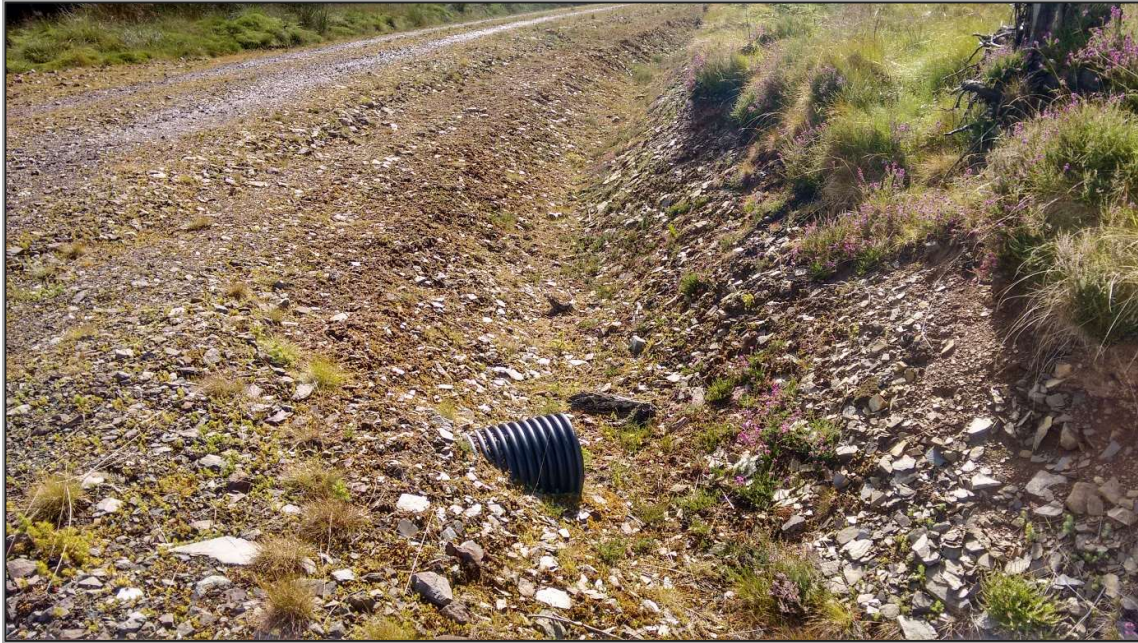
Plate 3-3: Example Swale and Cross Drain Serving Access Track
