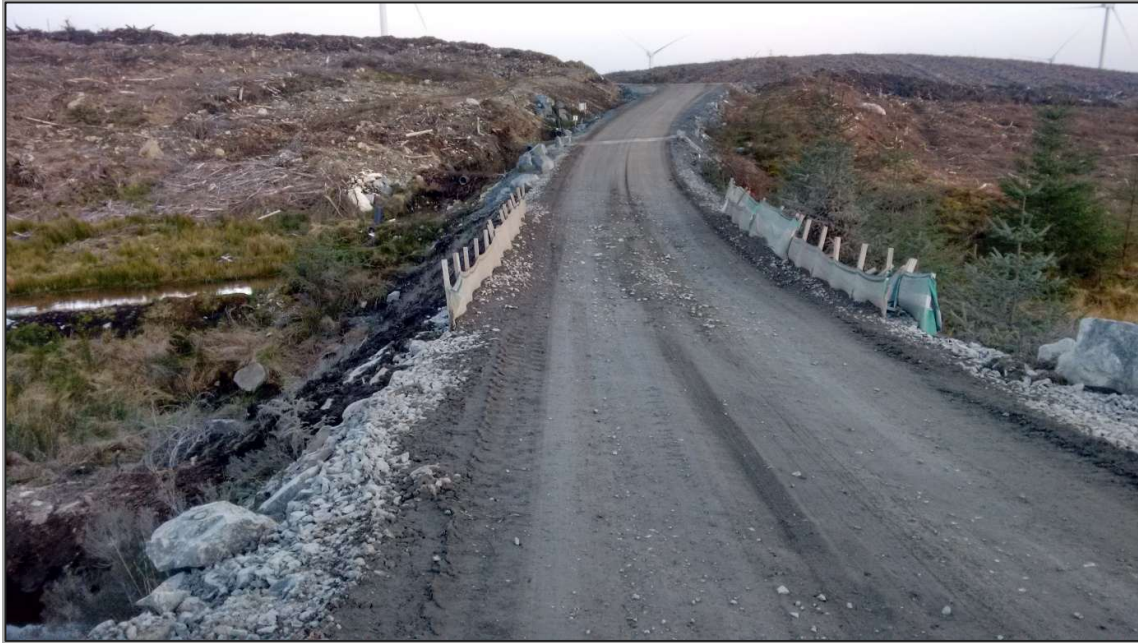
Plate 3-6: Example of Silt Fences at Watercourse Crossing
