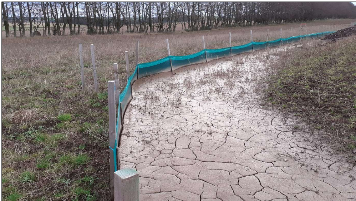
Plate 3-5: Example of Silt Fencing Around the toe of Soil Stockpile
