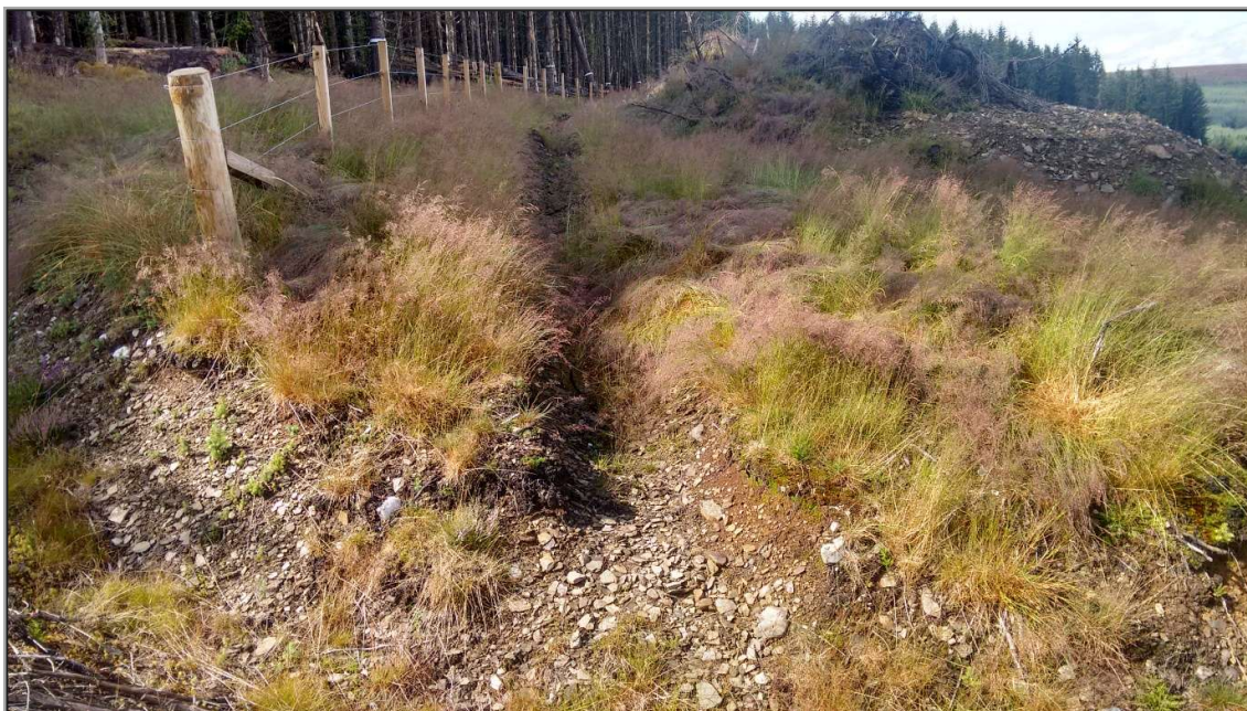
Plate 3-1: Example of Clean Water Diversion Ditch
